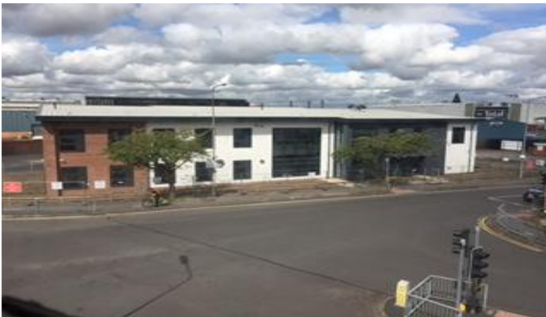
The New Medi-Centre, Warrington. Completed - August 2016. Full GP healthcare services commence - 8th of September 2016
