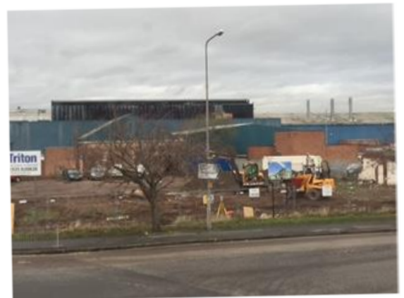
Tanners lane site Demolition- Dec 2015
